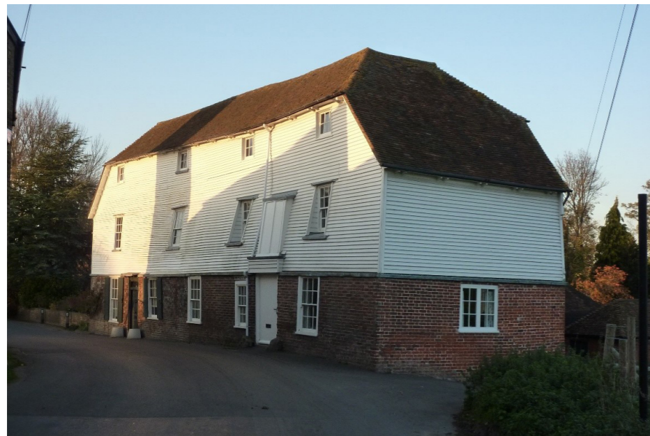
Figure 3.9 The mill house from the south.
