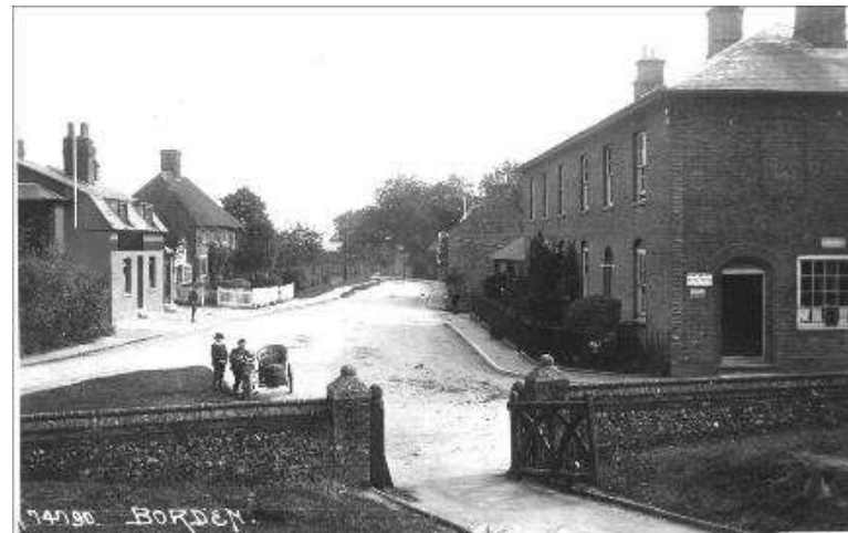
c.1900 view eastwards down The Street from the Churchyard
